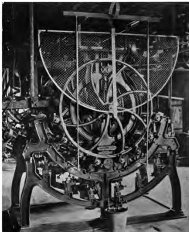
Fig. 3. Guard (raised) for Color Printing Machine.†
